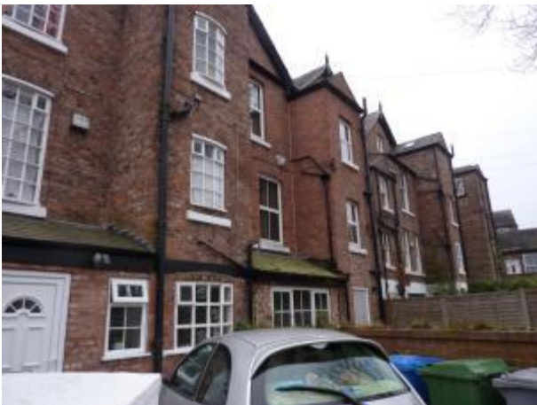
Photograph 36: Rear of Osborne Terrace, 17-23 Hale Road
