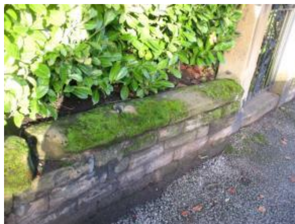
Photograph 13: Stone Wall with Evidence of Railings
