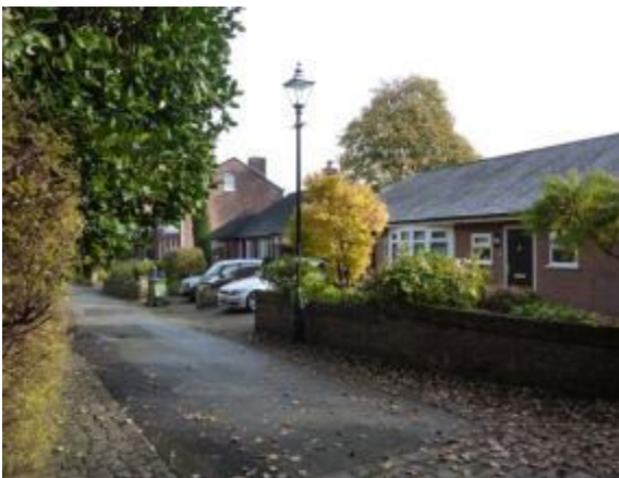
Photograph 10: Setts and Streetlamp on Lyme Grove
