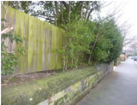
Photograph 50: Partial Loss of Screening Planting of Fence
