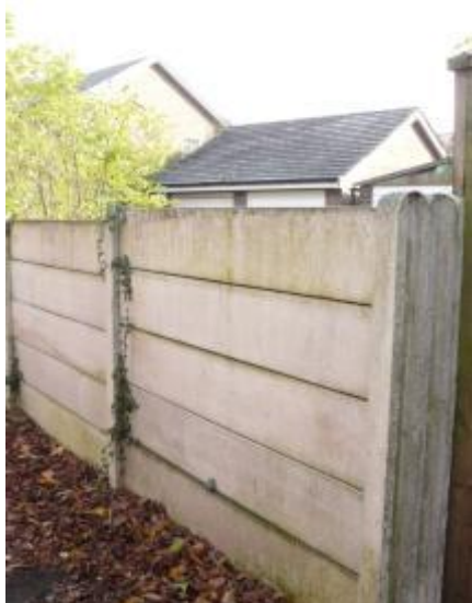
Photograph 44: Intrusive Concrete Fence on The Narrows
