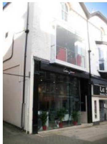
Photograph 41: Inappropriate First Floor Window
