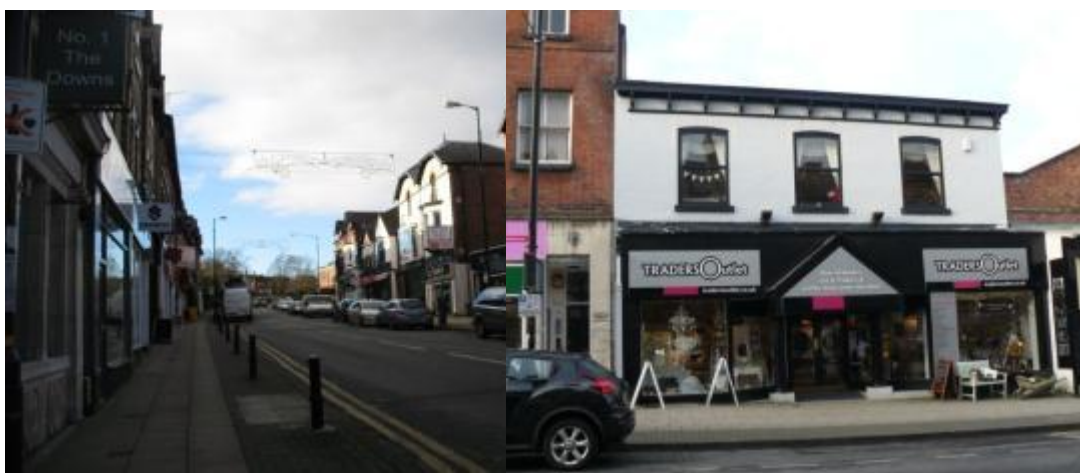
Photograph 48: Poor Repair, Wide Yellow Lines and Bollards, as well as Tall Streetlamps
