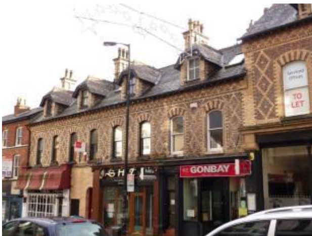
Photograph 40: Intrusive Permanent Awning
