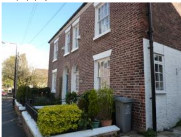
Photograph 12: Town Garden with Boundary Wall and Railing
