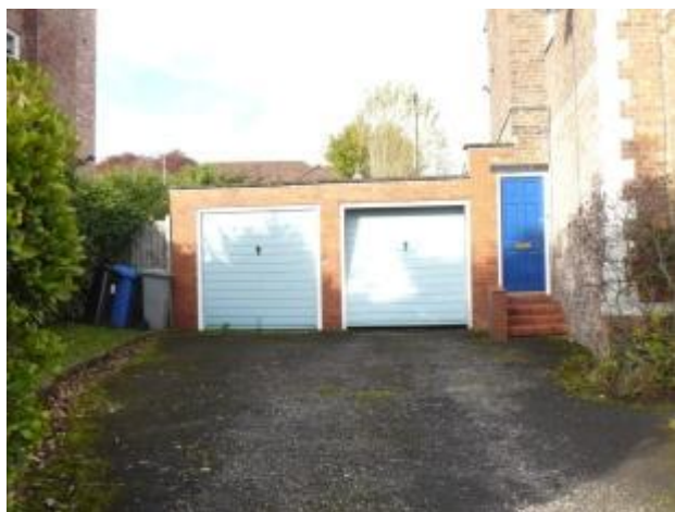
Photograph 42: Intrusive Garage/Hard Standing on Lyme Grove (Wide Opening not Visible)
